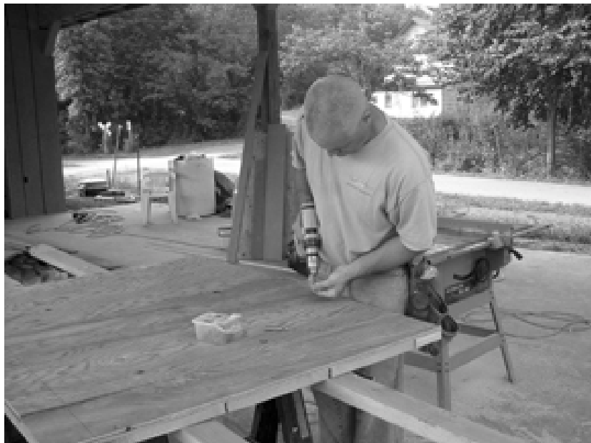
Tim Whitely of Westbank Contracting helping to build the pavilion
